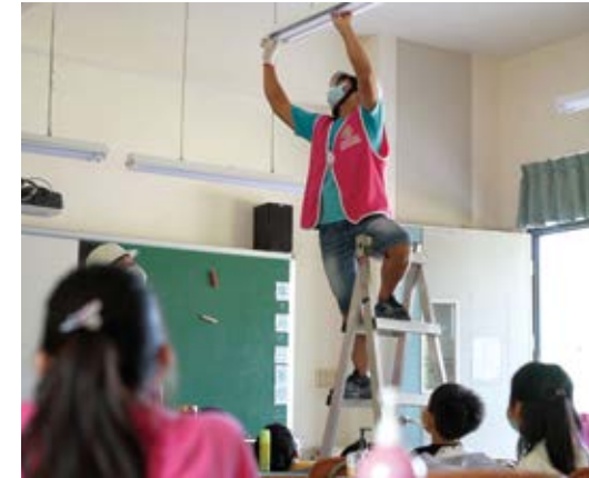
Campus LED installation projects
