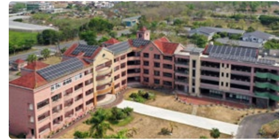
▶ Shanlin Junior High School Smart Microgrid Installation Project
